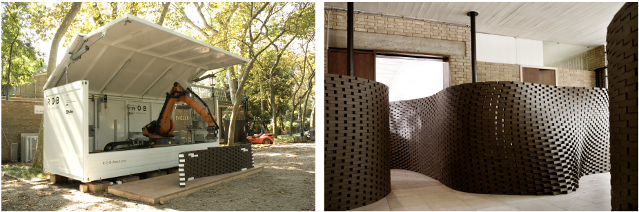
Fig. 2. left: On-site prefabrication performed with the R-O-B fabrication unit; right: Resulting in a highly articulated non-standard brick system at the 11th Venice Architectural Biennale (Gramazio & Kohler, ETH Zurich, 2008)
