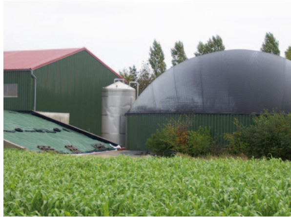
Fig. 7.4 Typical agricultural biogas plant in Germany using energy crops (corn) and other substrates as feedstock material. (Source: D. Rutz, WIP)
