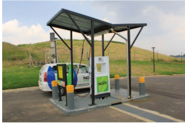
Fig. 15.4 Filling station of NOVO for upgrades landfill gas plant at the Sebenza landfill site. (Source: Hugo A., NOVO)
