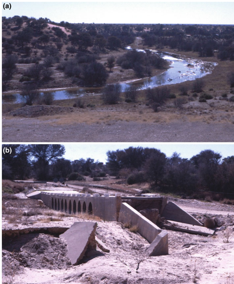
Fig. 15.2 The Kuruman River (a) in flood near Donkerdraai Farm in 1988, which caused considerable disruption to infrastructure including (b) the road causeway at Grootdrink Farm (Photographs D. Nash). See Fig. 15.1 for locations of images
