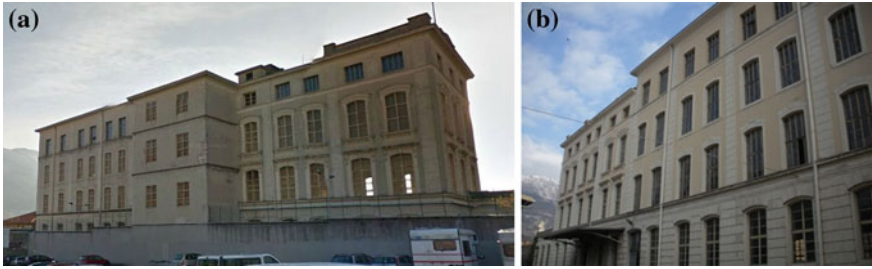
Fig. 2 a North-east facade. b North-west facade
