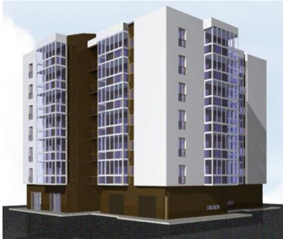
Fig. 22 Sunspaces with an entirely glazed shell (solution 2)
