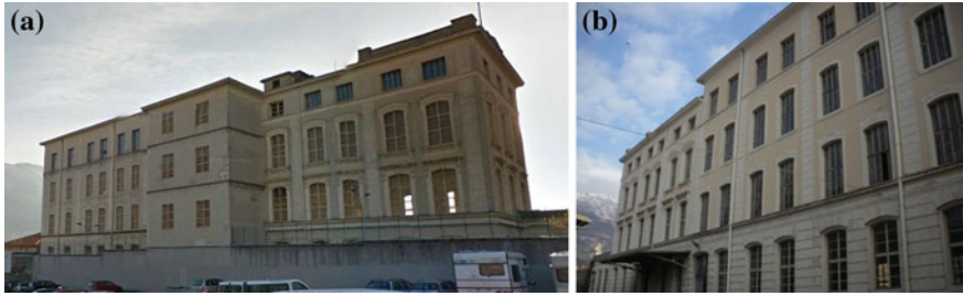
Fig. 2 a North-east facade. b North-west facade
