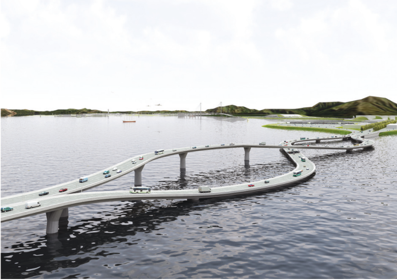
Fig. 7.2 Proposed “flipper bridge” between Hong Kong (left-hand traffic) and mainland China (right-hand traffic). Design by nl architects ( www.nlarchitects.nl ). Picture used with permission
