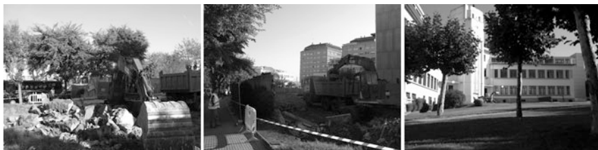
Fig. 8 Riazor. Removal of architectonic barriers (walls). Old School of Commerce ( right )
