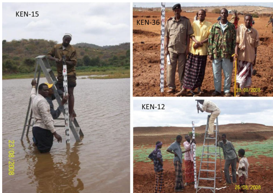
Fig. 5.4 Staff gauge installation efforts carried out in some of the Kenyan water points
