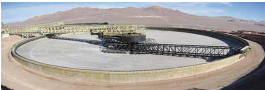
Fig. 8.14 125 m high-rate thickener (Smith 2013)
