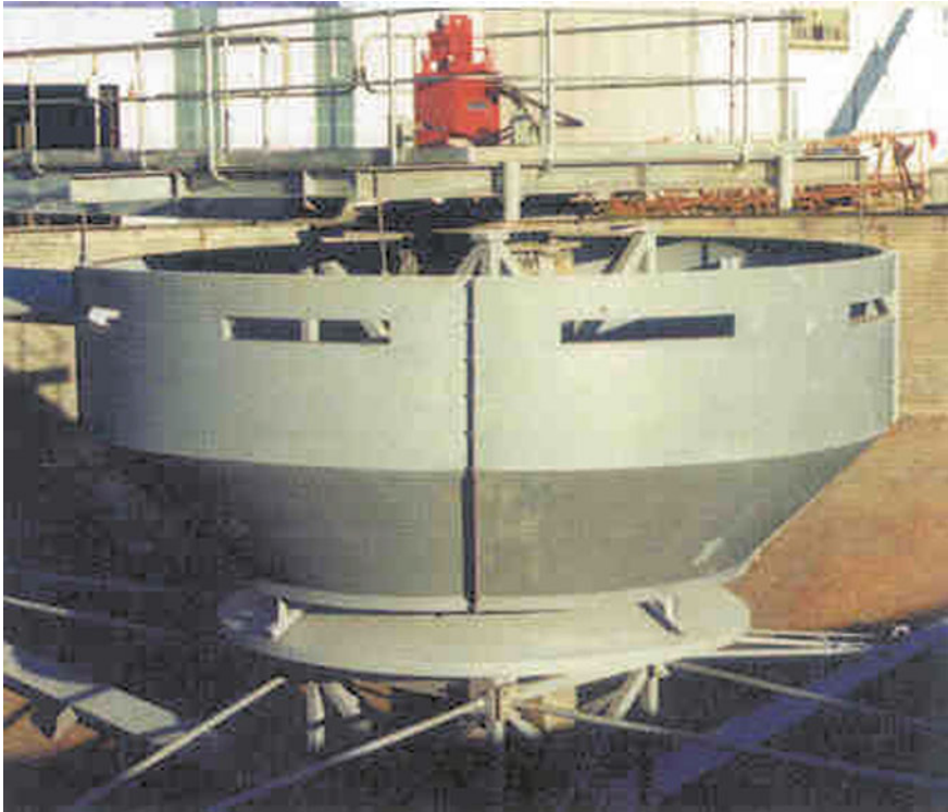
Fig. 8.100 Feedwell with water ports to dilute the feed (Supaflo technologies)
