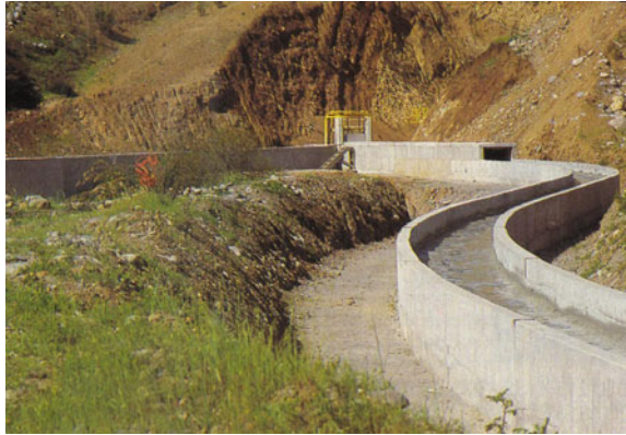
Fig. 1.10 Tailing channel in a Chilean copper mine
