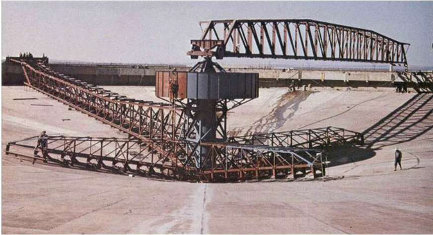
Fig. 8.7 Thickener with peripheral tracking system (courtesy of Eimco process equipment)
