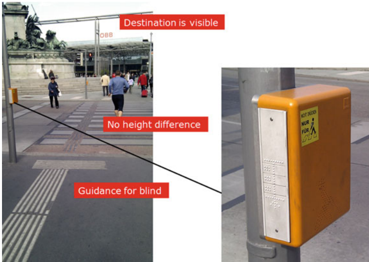
Fig. 5 Example of a crossing with visual and tactical guidance on different levels
