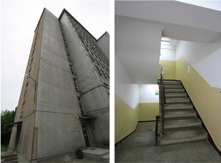
Fig. 1 Building and the staircase
