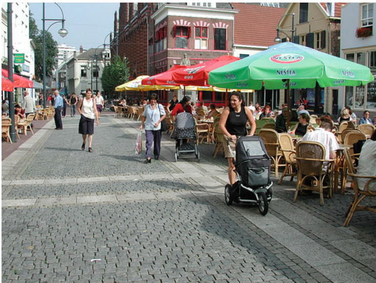
Fig. 7 Pedestrians like a smooth surface: the larger tiles are preferred by strollers. The pattern also gives a guidance for the terrace: till there and not further
