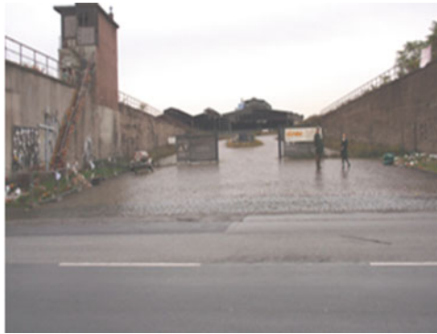
Fig. 6 Main access ramp (Photographed by one of the authors)
