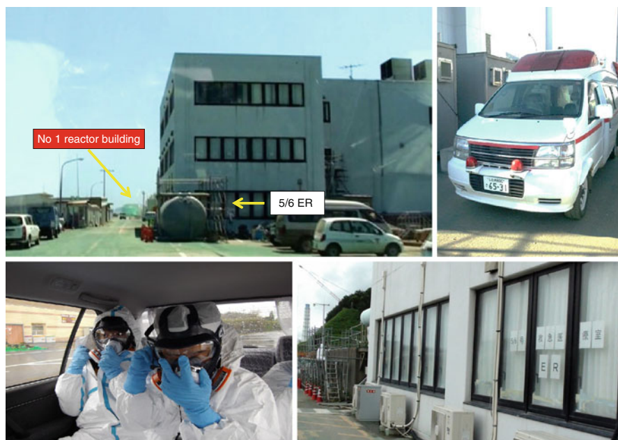
Fig. 3.17 Unit No 5/6 reactor Management building ( upper, left ) and 5/6 ER ( bottom, right ). Full PPE was required to reach 5/6 ER ( bottom, left ). Upper right is ambulance for emergency dispatch and transportation
