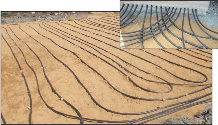
Fig. 5. Installation of the horizontal exchanger
