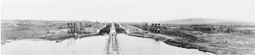
Fig. 13.13 Photograph taken in 1913 showing the Panama railway, the steam shovels, and the locks in the Panama Canal project
