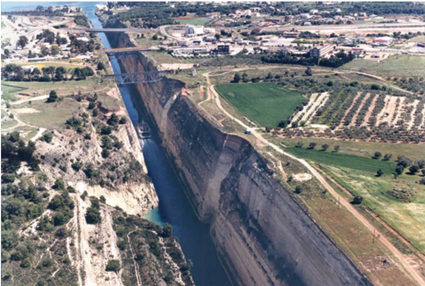
Fig. 13.11 Aerial photograph of the Corinth Canal
