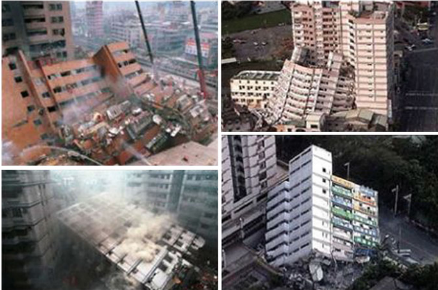
Fig. 13.35 Photos of buildings collapsed by the Tōhoku earthquake
