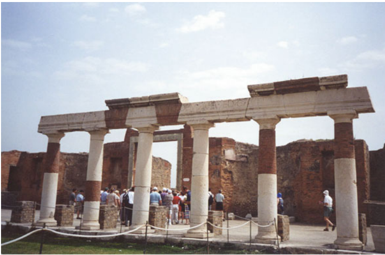
Fig. 11.16 Reconstruction of columns in the forum at Pompeii. Note the angular cuts in the beams mounted above the columns
