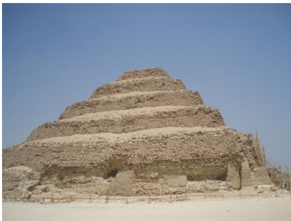
Fig. 1.4 Djoser's step pyramid. Note formwork on the right
