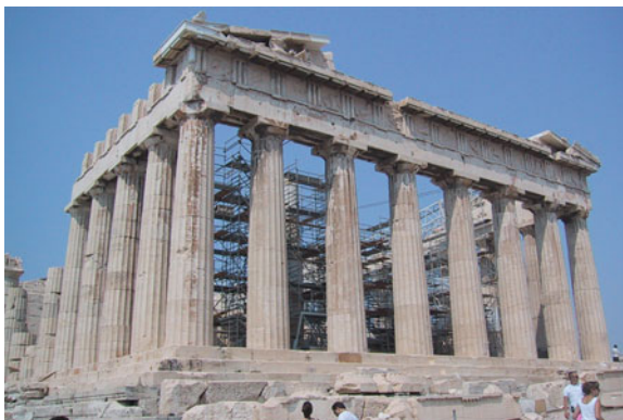
Fig. 2.3 Photograph of the Parthenon. Note the renovations underway
