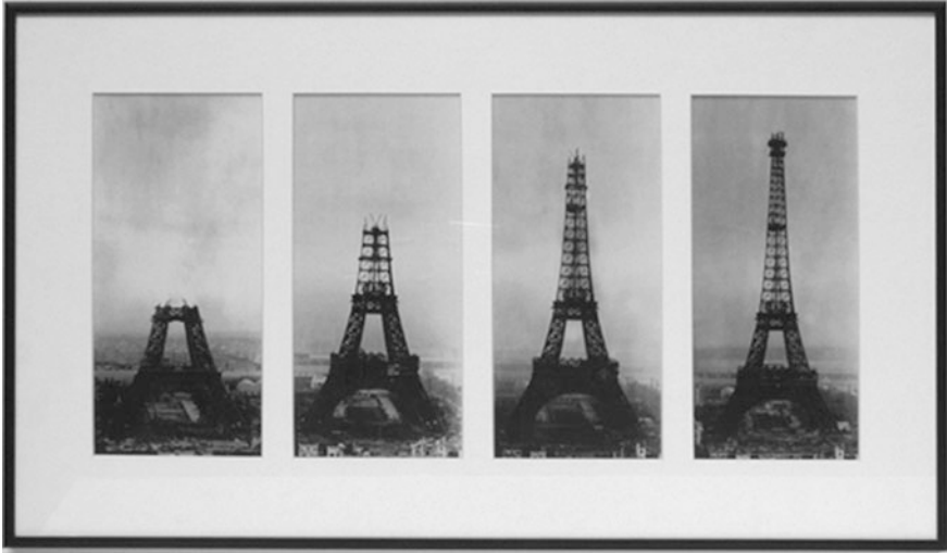
Fig. 9.33 Photographs of the Eiffel Tower during construction
