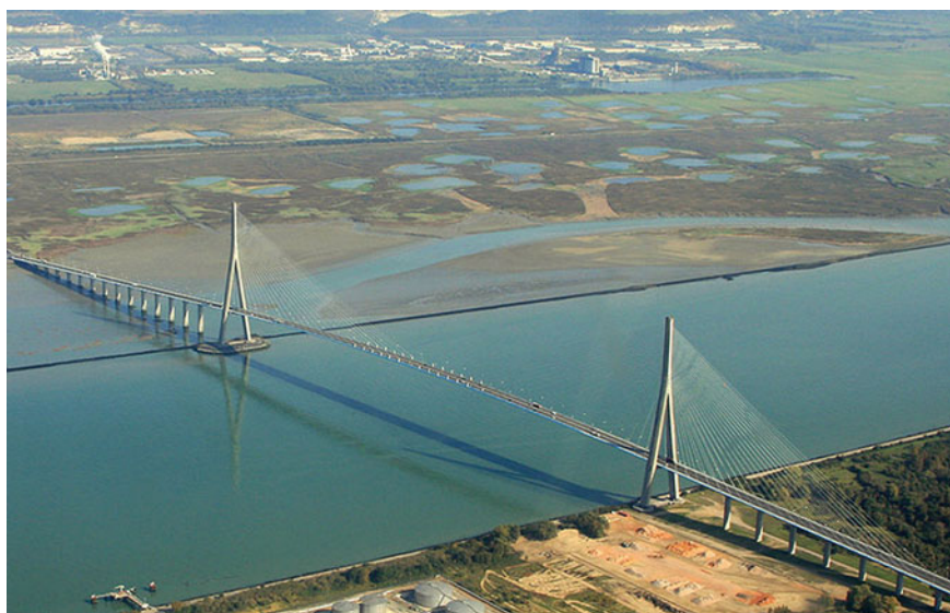
Fig. 9.42 Photograph of the Pont de Normandie
