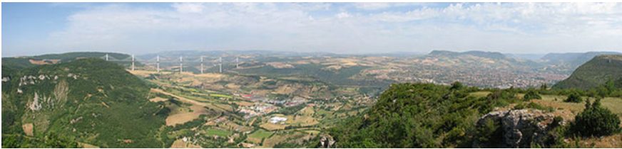
Fig. 9.44 Photograph of the Millau Viaduct in Southern France
