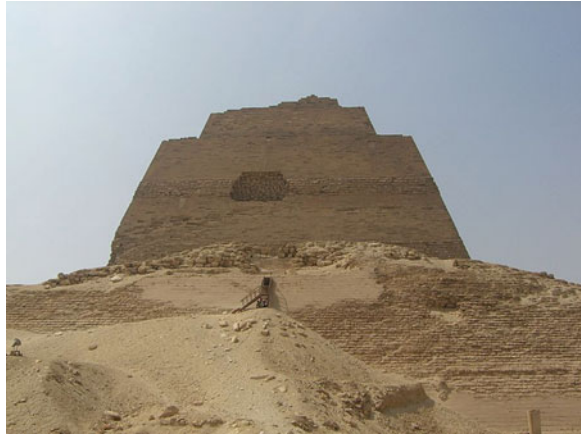
Fig. 1.5 Snefru's failed meidum pyramid. Note the rubble pile in the foreground
