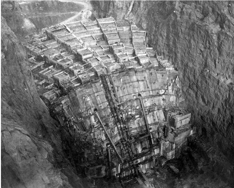
Fig. 13.19 Photograph showing the formworks for the massive concrete columns in Hoover dam
