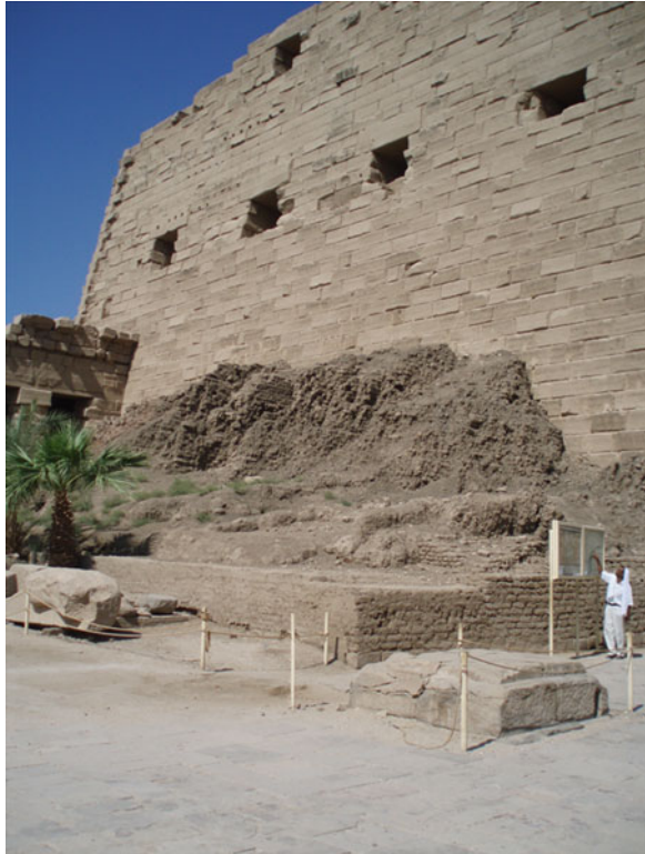
Fig. 1.10 Photo of the entrance gate of the temple of Karnak. Note remnants of the mud brick ramp
