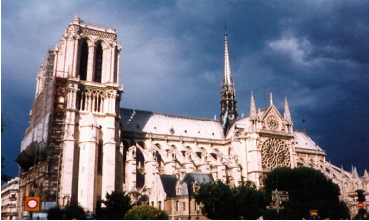
Fig. 4.14 Photo of Notre Dame Cathedral in Paris. Note the flying buttresses deployed along the nave and the choir, as well as the bell tower, all constructed for structural purposes
