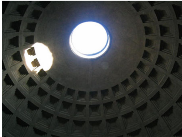
Fig. 3.15 The Oculus in the Dome of the Pantheon. Note the inlaid pattern in the concrete ceiling
