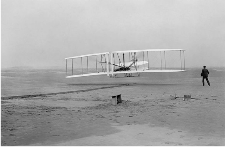
Fig. 12.9 The first manned flight of a heavier-than-air vehicle on December 17, 1903
