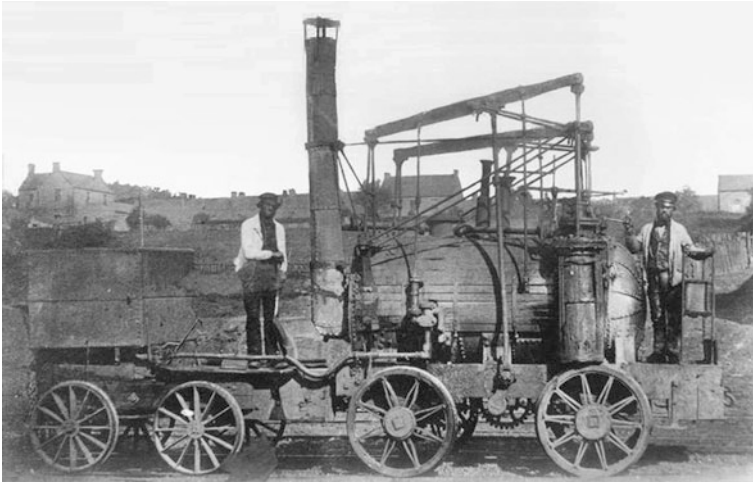
Fig. 12.2 Photo of the puffing billy—an early steam locomotive
