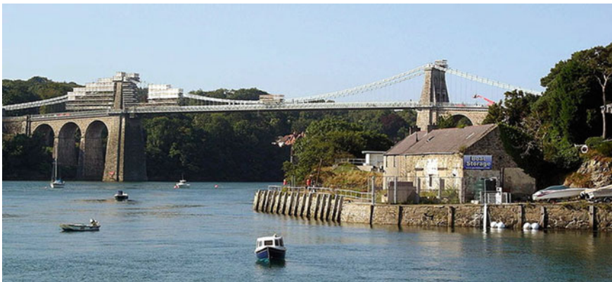
Fig. 9.30 Photograph of the Menai Suspension Bridge
