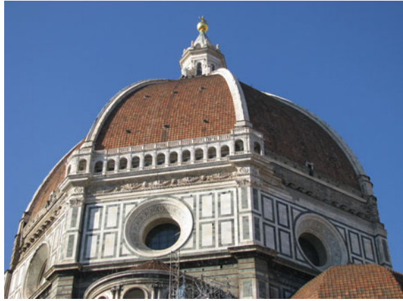
Fig. 5.9 The Brunelleschi Dome in Florence. Note the octagonal shape
