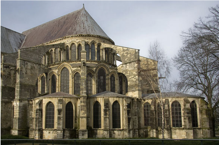
Fig. 4.12 Early Flying Buttress (c. 1170) attached to the Choir of the Cathedral of St. Remi in Reims
