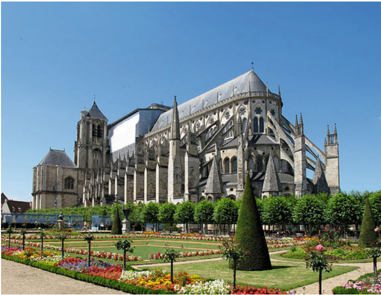
Fig. 4.13 Multi-tiered Flying Buttresses attached to Bourges Cathedral. Note the massive bell tower at the far end of the cathedral
