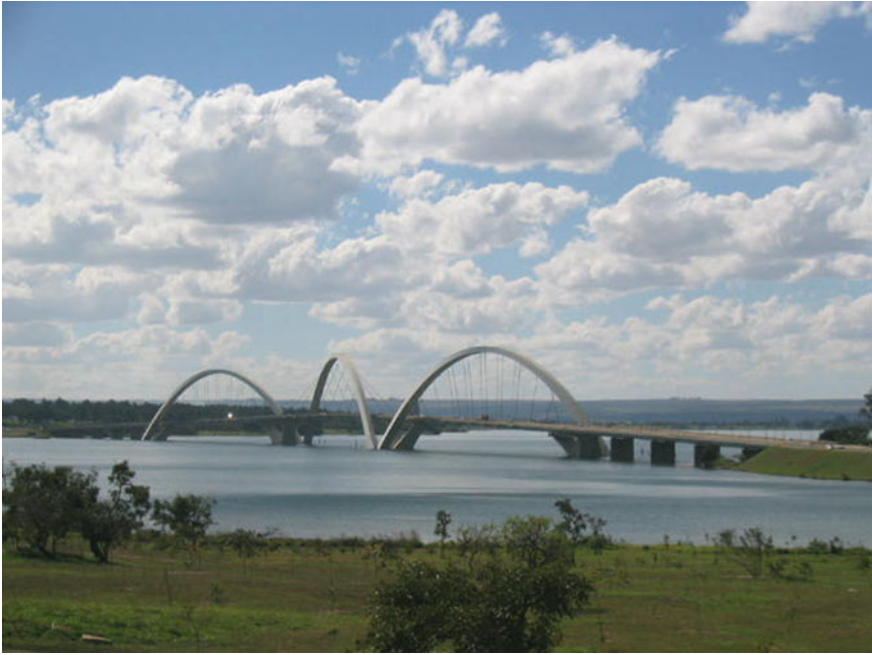
Fig. 9.43 Photograph of the Jucelino Kubitschek Bridge
