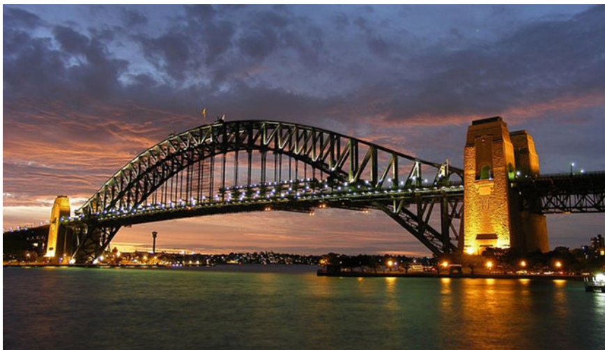
Fig. 9.41 Photograph of the Sydney Harbor Bridge
