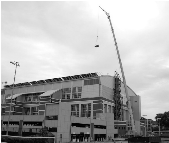
Fig. 2 Boom Crane Working on the Olympic Pool
