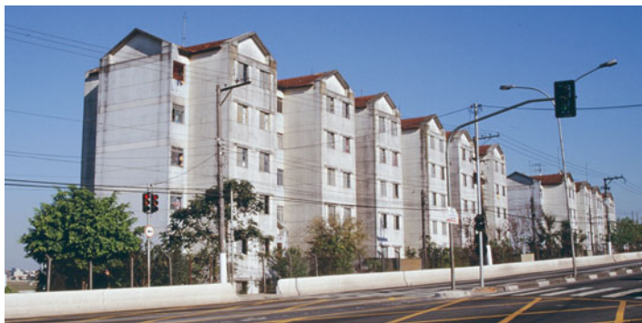
Photo 4.10 Favela Sul – Cingapura apartments
