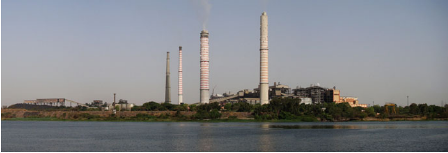
Fig. 20.8 Hydroelectric thermal power plant at Kota. Courtesy: Sunil Singhal, Kota
