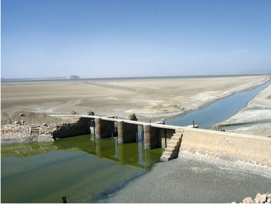
Fig. 8.6 Good rainfall in the year 2010 led to influx of salty water from the main lake to the reservoirs via sluice gates. Courtesy: Dr. Seema Kulshreshtha
