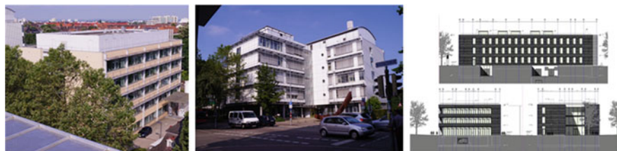
Fig. 7 The Institute of Macromolecular Chemistry ( left ), the Freiburg Materials Research Center, FMF ( center ) and the new Freiburg Institute for Interactive Materials and Bioinspired Technologies (FIT), which is currently under construction
