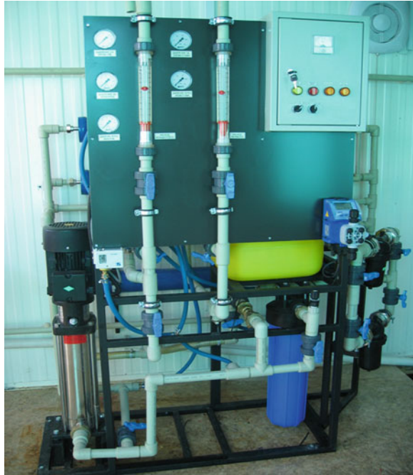
Fig. 2 Reverse osmosis water treatment produced by LLC “Membrane technologies”
