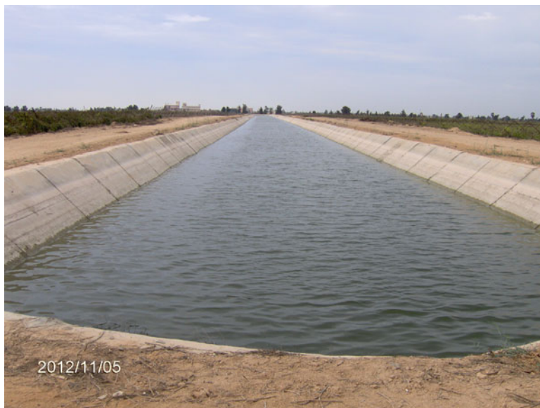
Fig. 8 The main irrigation canal is lining in Nubaria district, Egypt because of the very high infiltration rate or low soil water retention of sandy soils. Drip and sprinkler irrigation are common in this area (Photo by H. El-Ramady)
