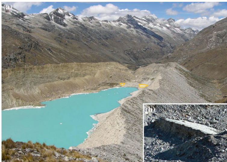
Fig. 5 View on lake Palcacocha with two artificial dams ( highlighted by the orange line ); steep nearly vertical lateral moraines are visible on both sides surrounding the lake. The detail picture (Part b ) was taken after the 2003 event and captures the damaged artificial dam
