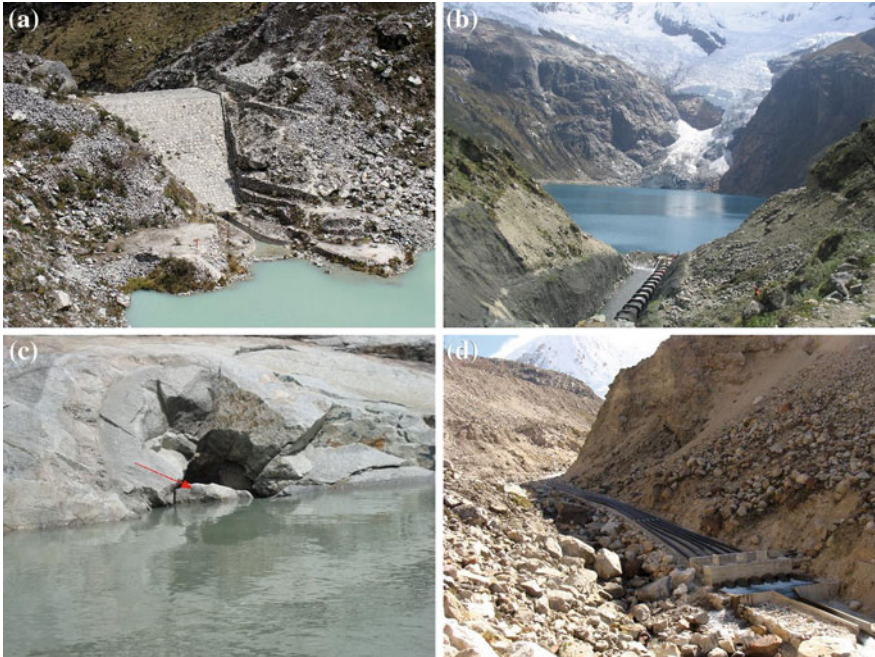
Fig. 9 Examples of remedial works. Part a shows artificial dam and concrete outlet of lake Llaca in the central part of the Cordillera Blanca; dam freeboard is 12 m. Part b captures ongoing work on the dam of lake Rajucolta in 2004. Part c shows the entrance to the tunnel excavated in the bedrock dam of lake No. 513 ( red arrow ). Part d shows six siphons installed in fall 2011 to drain and lower the water level of lake Palcacocha
