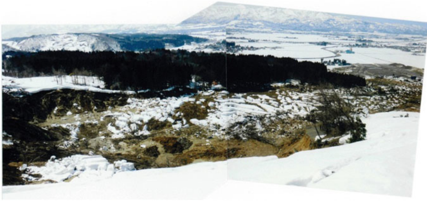
Fig. 2 Overview of the landslide area showing the head scarp
