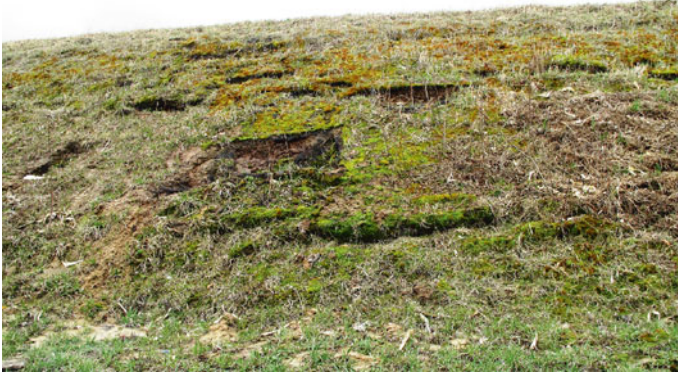
Fig. 12 The creep deformation of the slope bottom (K560+700 section)
