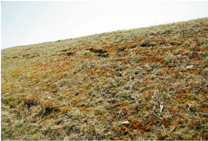
Fig. 13 The crack in the middle of the slope (K560+700 section)
