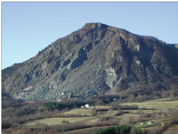
Fig. 12 Mt. Beni after the main collapse on December 28, 2002
