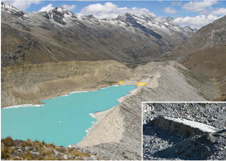
Fig. 5 View on lake Palcacocha with two artificial dams ( highlighted by the orange line ); steep nearly vertical lateral moraines are visible on both sides surrounding the lake. The detail picture (Part b ) was taken after the 2003 event and captures the damaged artificial dam
