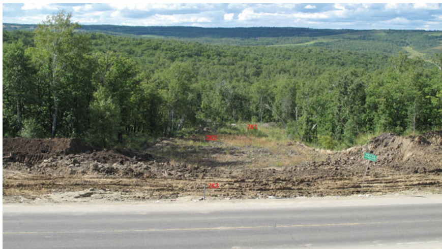
Fig. 3 K178+530 landslide photo
