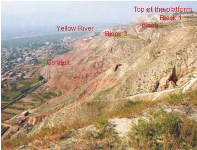
Fig. 5 The Huangci landslide at the south side of the Heifangtai platform
