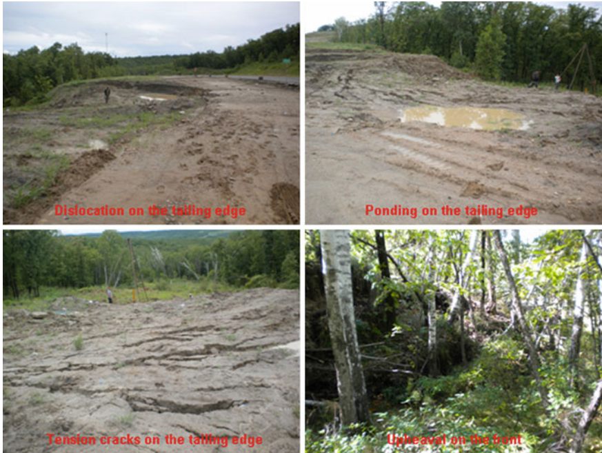
Fig. 3 Landform characteristics of the K178+ 1 530 landslide
