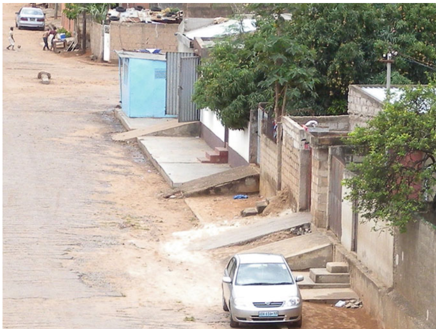
Fig. 13.3 Maputo, KaMaxakeni district, 2 Nov. 2011. The raised entrances of building plots constructed to exclude floodwater (Tiepolo 2011)
