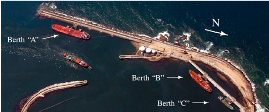
Fig. 1 Leixões Oil Terminal, Porto, Portugal
