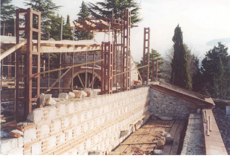
Fig. 8.10 The church during reconstruction
