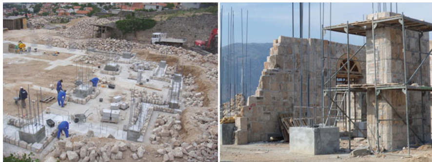
Fig. 8.26 Beginning of the construction of the church in May 2011
