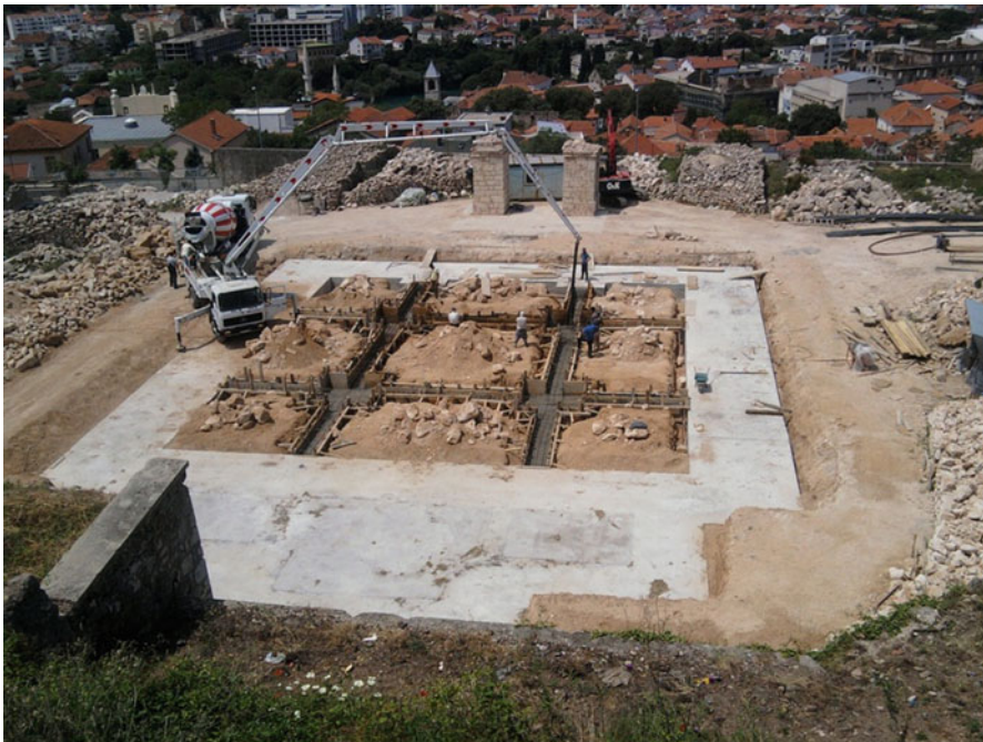
Fig. 8.20 Newly designed RC foundation in the course of construction
