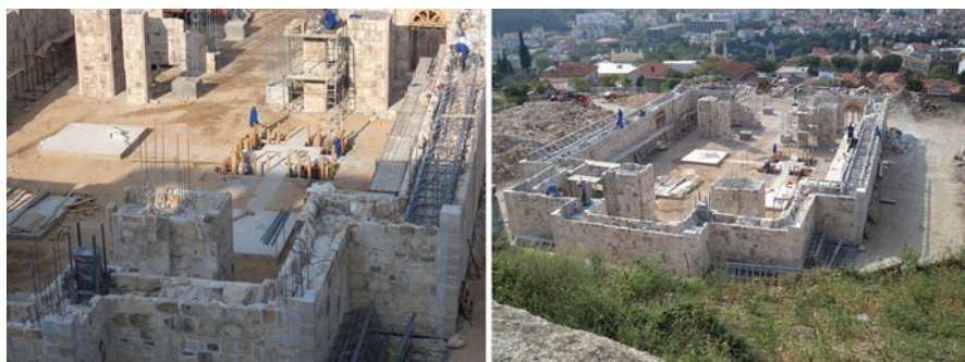
Fig. 8.27 Construction of the church up to the level of first horizontal ties
