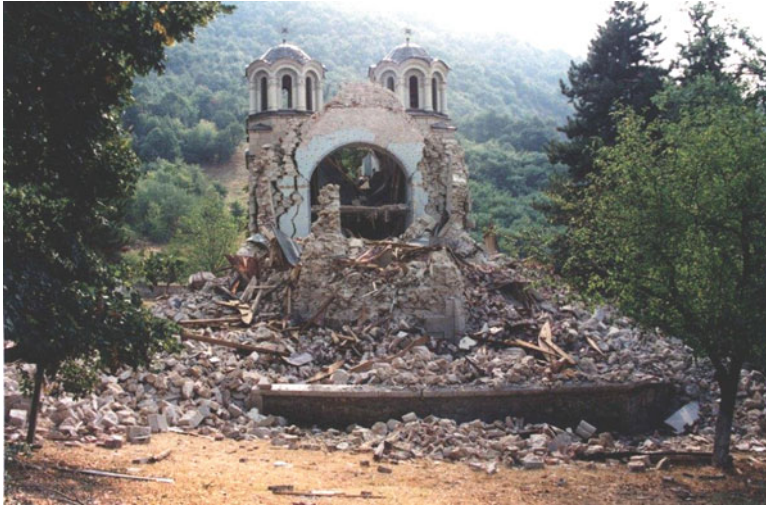
Fig. 8.13 The church after detonation
