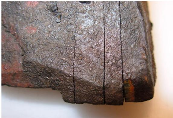
**Fig. 12** Intersecting floor cracks indicative of upward heave of the slab
