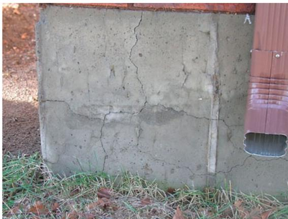
between 5 and 10 % pyrrhotite, pyrite and chalcopyrite, all sulphides of iron. Domestic house construction typically uses concrete with compressive strengths of 20–25 MPa for foundation and basement wall construction. The source quarry for the coarse aggregate was a small local quarry that only operated for a few years.
