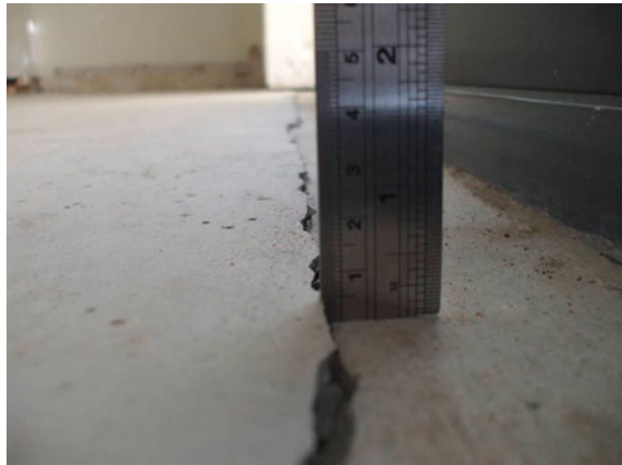
Fig. 16 Ground floor slab adjacent to patio doors, before and after expansion of the stone fill
