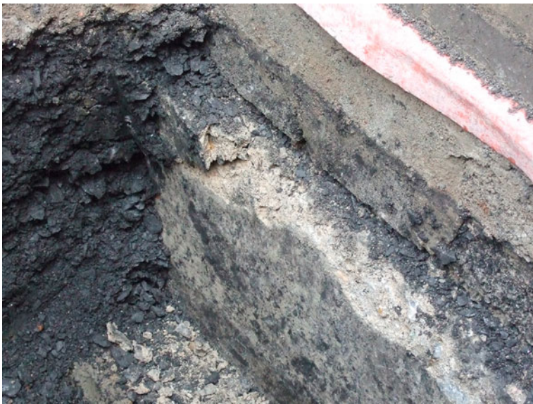
Fig. 28 Deterioration of concrete at the top of the beam, TP 11, and the nature of the dark deleterious fill adjacent to it
