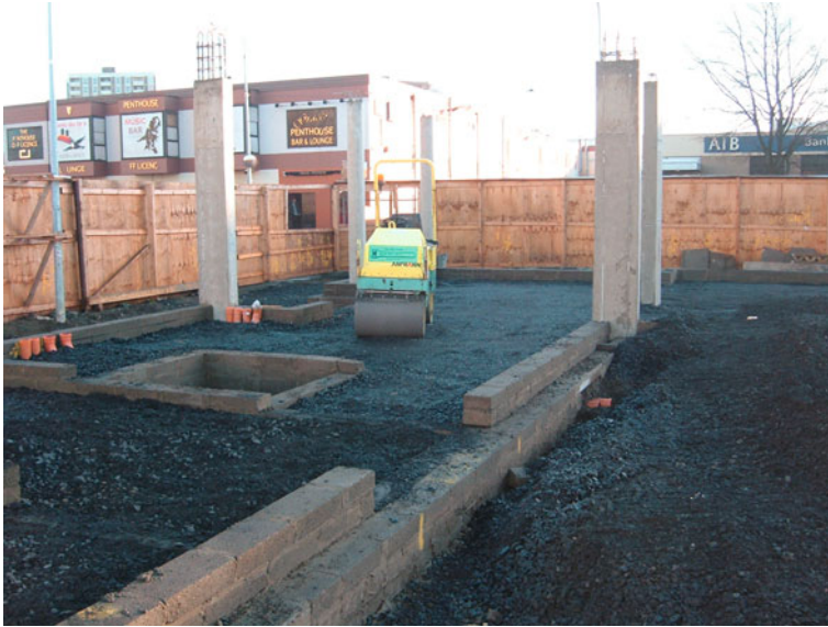
Fig. 5 Fill being compacted by roller, December 2004
