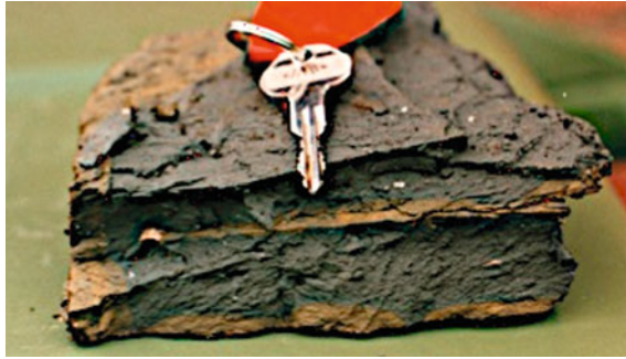
Fig. 10 Oxidation along discontinuities in the London Clay
