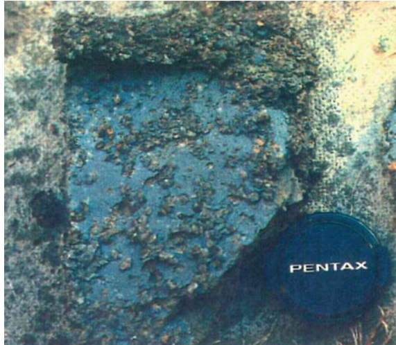
Fig. 47 Isolated gypsum crystals on Lias Clay exposed during the investigations
