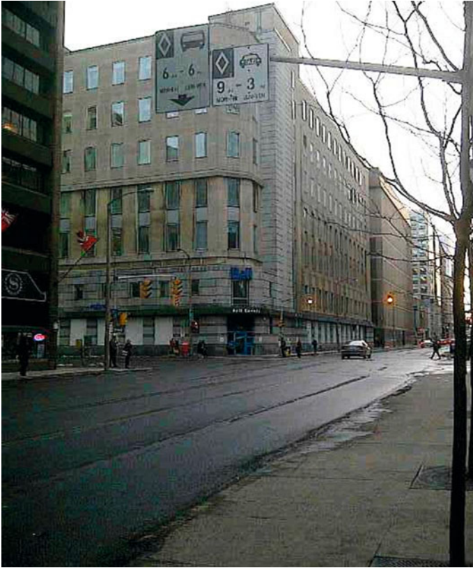
Fig. 2 Bell Canada Building, Albert Street, Ottawa
