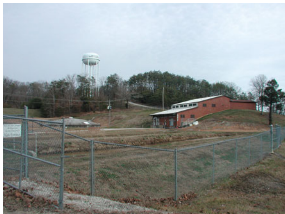
Fig. 29 Clay City (Beech Fork) Water Treatment Plant
