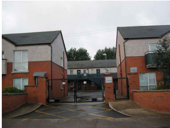
Fig. 1 View from Clancarthy Road into the development
