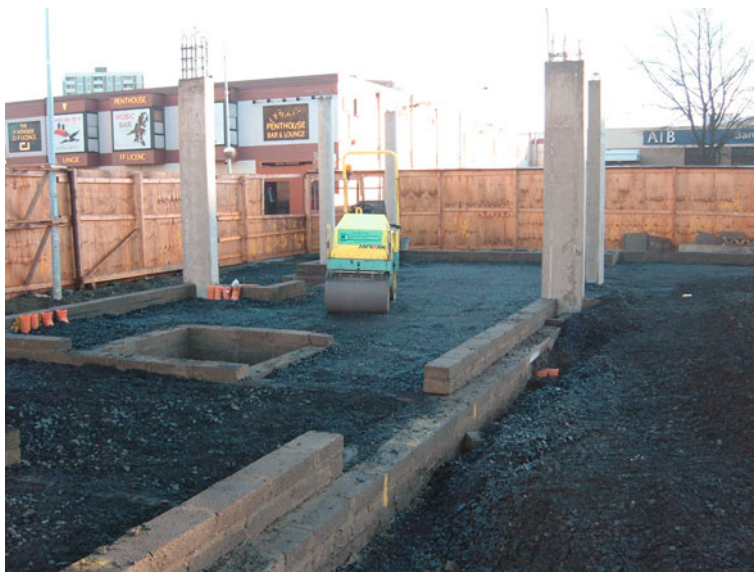
Fig. 5 Fill being compacted by roller, December 2004
