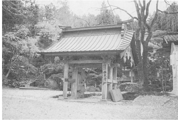
Fig. 23.6 Saiko-temple gate with a projecting horizontal crossbeam from Catalog for Kesen daiku ten
