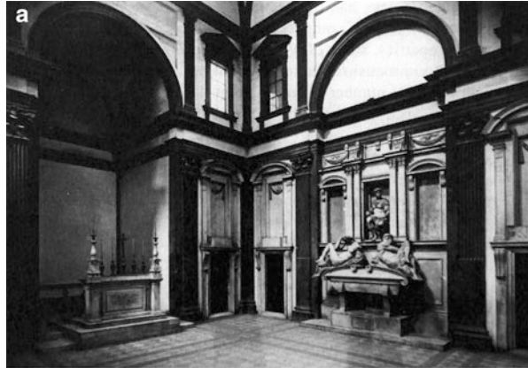
Fig. 37.10 (a) Interior of the Medici chapel. Photo: Kim Williams (b) Plan of the Medici chapel. Drawing: Kim Williams
