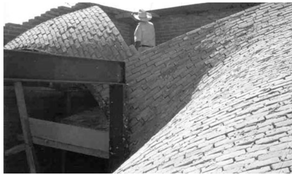
Fig. 21.6 Vaults built to cover a flat area limited by a rectangular or square perimeter. Photo and drawing: authors
