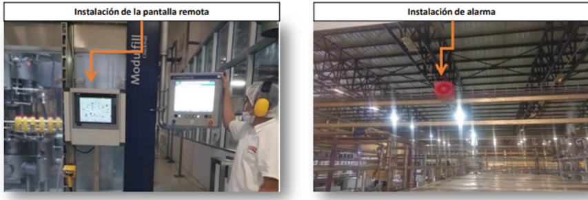
Fig. 8. Installation of remote screen and alarm in the pasteurization machine
