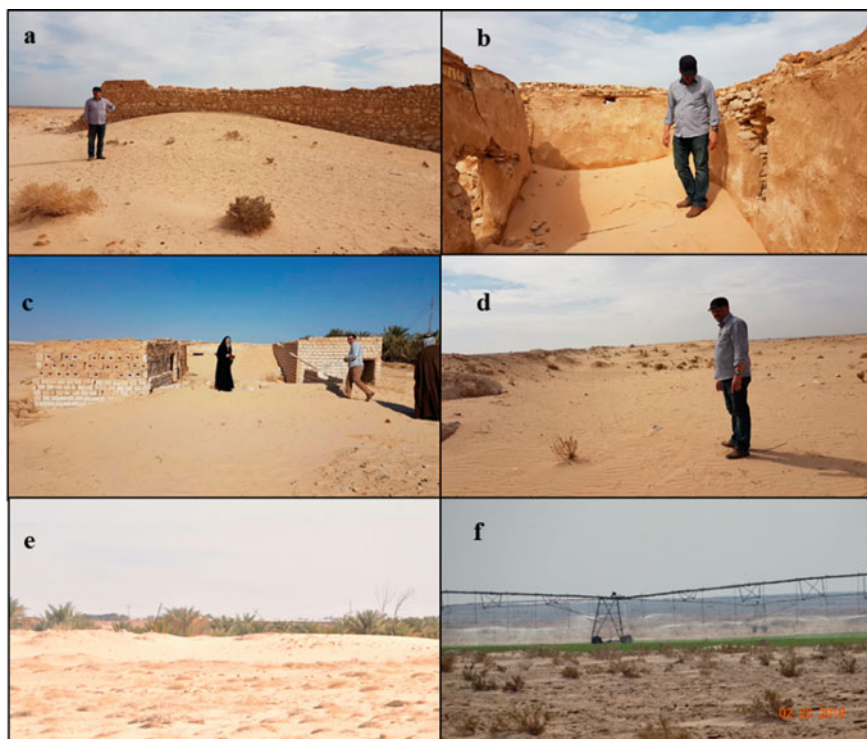
Fig. 15 a and b Houses covered by sand in the Al-Ruhba area; c Houses covered by sand in the Al-Rahima area; d Irrigation channel filled with sand; e and f Farms surrounded by Nabkha and longitudinal dunes
