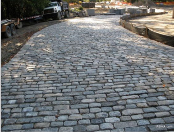
Fig. 3.96 Typical cobblestone road
