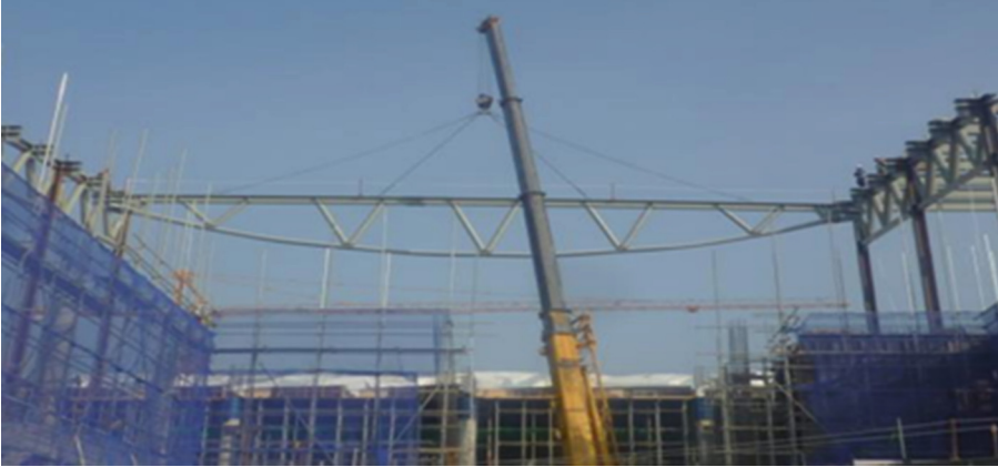
Fig. 1. Combined steel truss with a span of 30 m [17]
