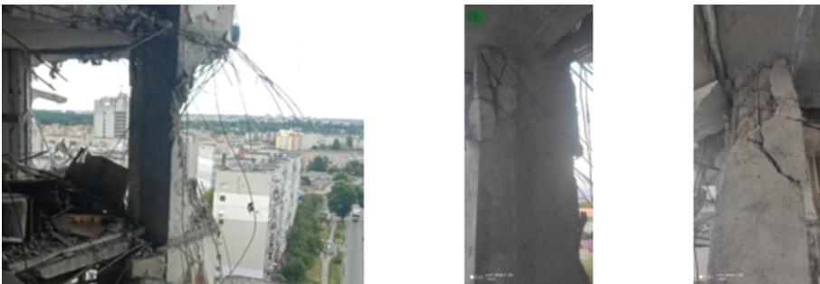
Fig. 1. Pylon at the first stage of work. (Photo Oleh Tabarkevych).
