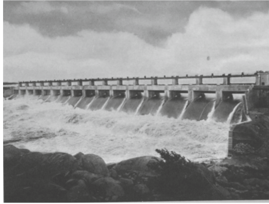
Fig. 14. A free roller gate built in India in 1932 by Glenfield & Kennedy [25]
