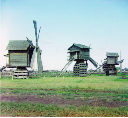
Fig. 3. Post mills in 1912 in Siberia (Source: Wikipedia)
