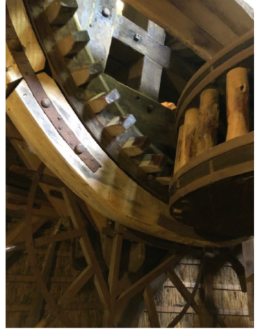
Fig. 21. Brake wheel and pinion in the cap of the mill in Laren. The blocks of the Flemish brake are clearly visible.
