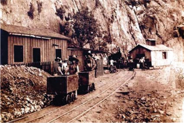
Fig. 9. Steel carts and tracks for moving minerals outside the mine ( https://cienciauanl.uanl.mx/?p=4176 )
