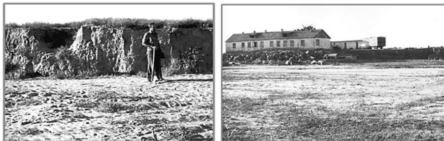
Fig. 10 Erosion of loess banks after the first year of reservoir's filling ( left ) and destruction of buildings on the bank ( right ) in 1967 ( photo by V.M. Starodubtsev )
