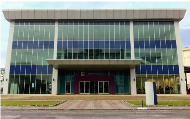
Fig. 2 PTAR library building
