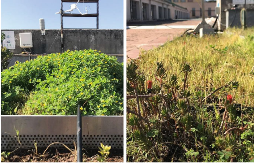
Fig. 8.5 An experimental blue-green roof on the building of the engineering department of the University in Palermo (Italy) investigated by Pumo et al. (2023) (Author's photo)
