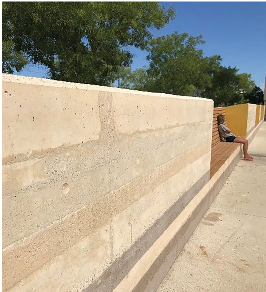
Fig. 10.5 Rammed earth concrete wall with golden niches. (Source: L+P 2020)
