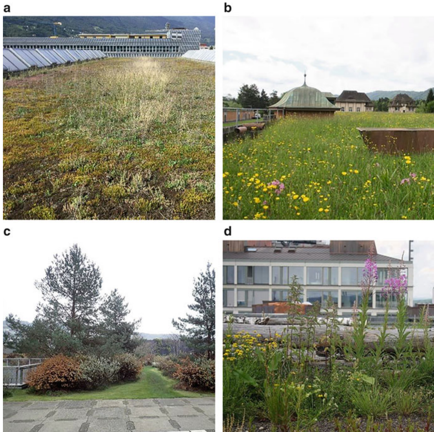
Fig. 8.2 Examples of different types of green roofs in Switzerland: (a) the extensive green roof of the ex-Swisscom building in Giubiasco (Author's photo), (b) the semi-intensive green roof of the water filtration plant in Wollishofen, Zurich (Author's photo), (c) intensive green roof of the Toni Areal campus in Zurich (Author's photo), (d) biodiverse green roof of the Baufeld C in Zurich (Author's photo)
