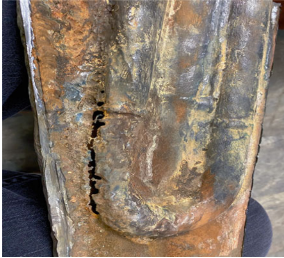
Fig. 2 Sulphur dioxide dewpoint corrosion of boiler tube due to ingress air
