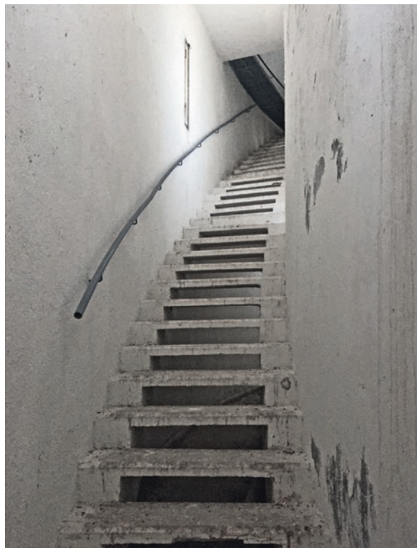
Fig. 16.7 Helicoidal concrete stairway, located between the external and the internal wall of the Water Tank. (© Nicola Panzini 2023)
