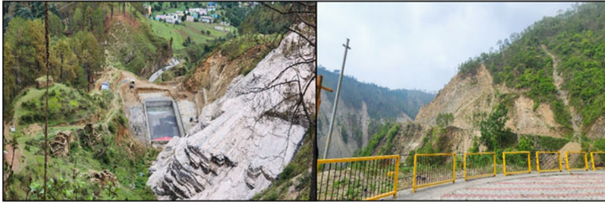
Fig. 8 Infrastructure development in the Indian Himalayan Region. Source Authors
