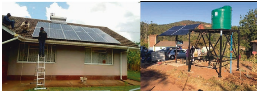
Fig. 8.3 Use of solar energy and water storage tanks at the home level. (Source: Authors 2019)
