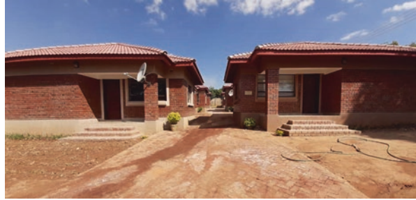
Fig. 8.2 Cluster houses demonstrating the implementation of densification. (Source: Authors 2019)
