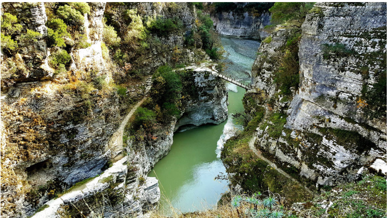
Fig. 7 Osum canyon and river, Zabërzan bridge
